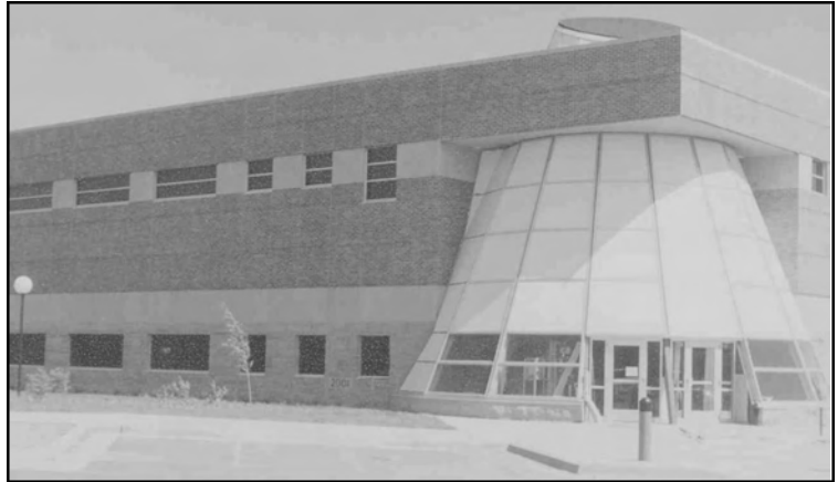
July 31, 2001 - The temporary panels are installed in the lobby area and the landscaping is complete.
